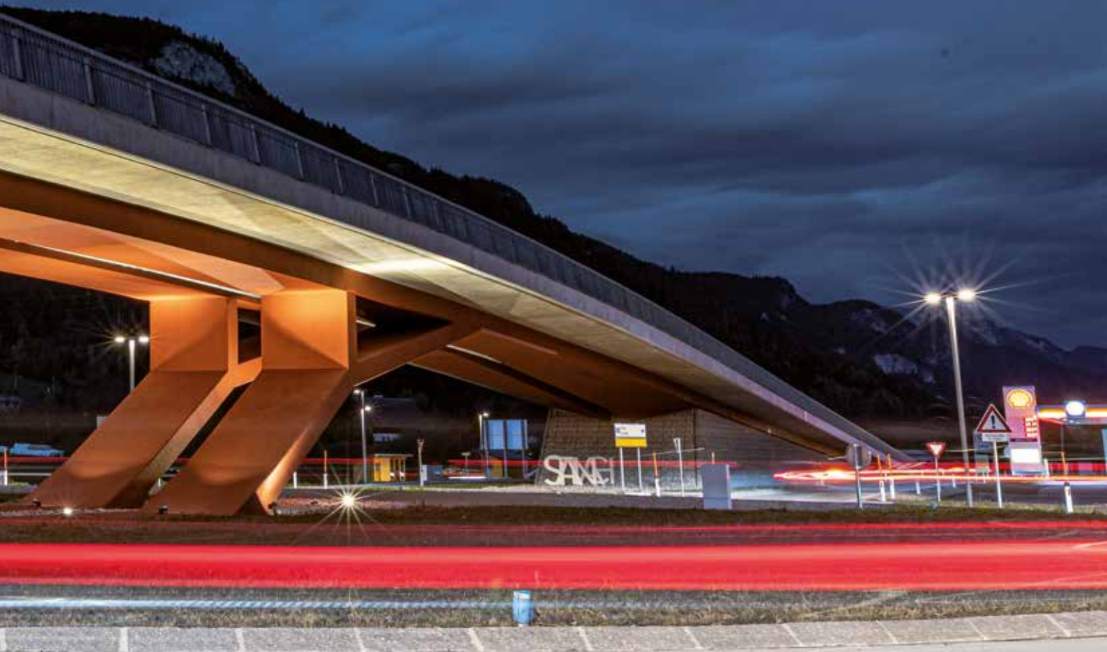
Most Grimmingbrücke, Trautenfels, Austria
